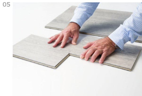
Press the planks gently while sliding
