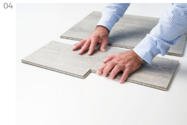
To disengage on the short side, slide the planks the opposite direction
